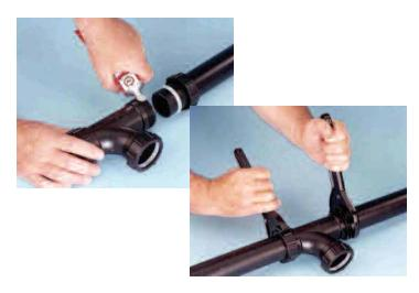
Loosely assemble the joint and proceed to hand tighten the knurled nut. Using two spanners further tighten the joint. The nut must be tightened to its full thread capacity.
